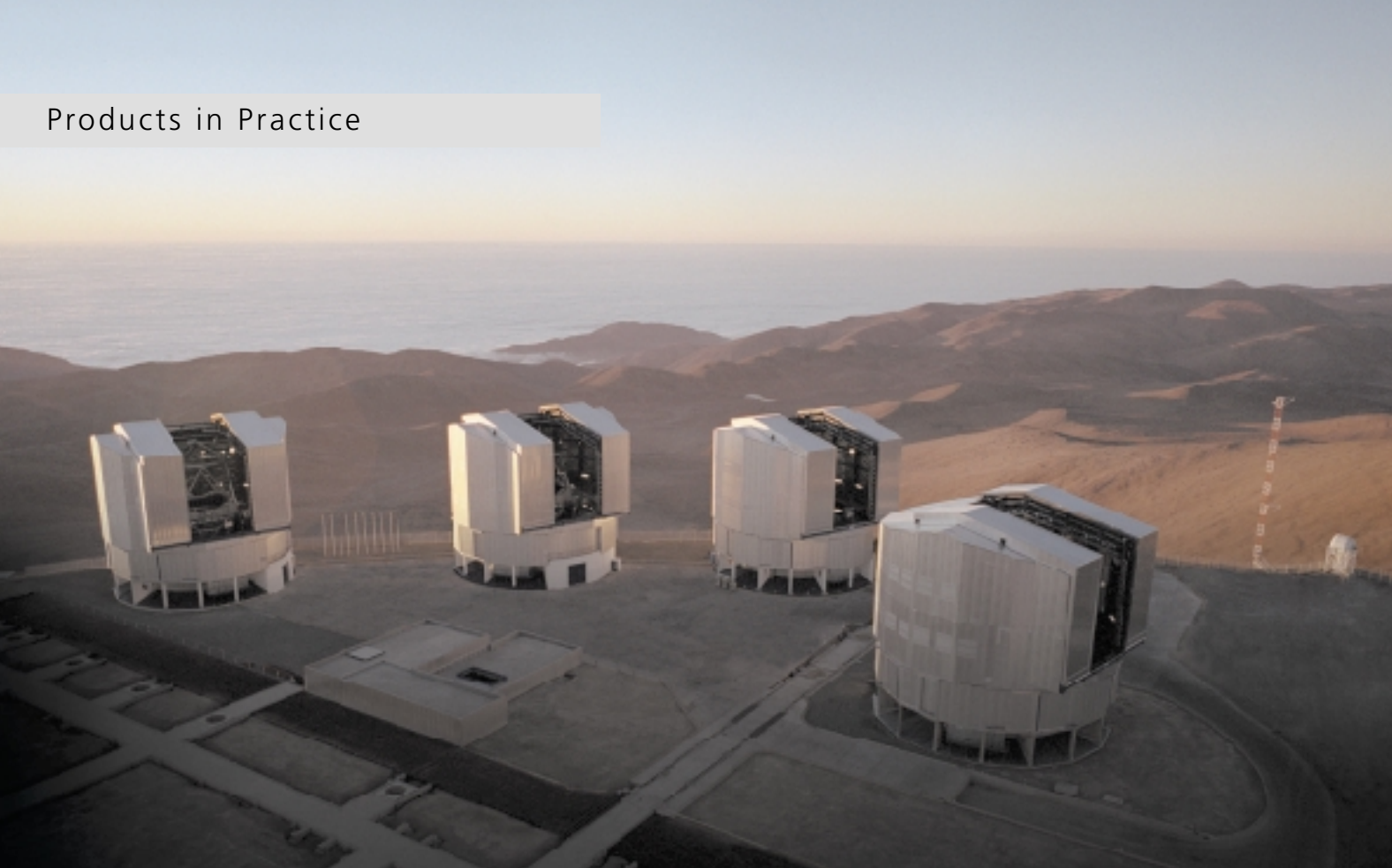
Fig. 5: An interferometer on Cerro Paranal will combine the light of two or more ESO telescopes in an underground tunnel, providing images of significantly increased resolution. The VLT will then be able to simulate a telescope with a mirror diameter of 200 m and will "see" up to 100 times more sharply than Hubble. Zeiss is manufacturing mirror units for this interferometer. (Photos 4 and 5: ESO).
